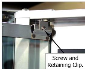
5. Lift the inner glass up onto the locking catch to lock into position.
